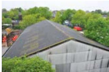
Figure 32 Asbestos cement roof and cladding
