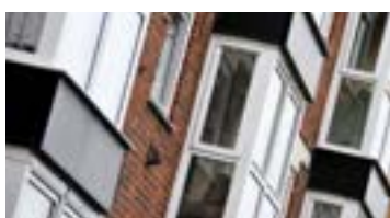
Figure 16 AIB exterior painted panel
