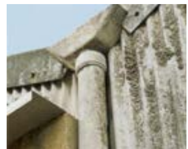
Figure 35 Asbestos cement downpipe
