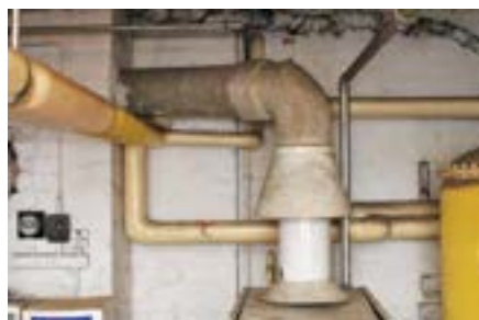
Figure 34 Asbestos cement boiler flue
