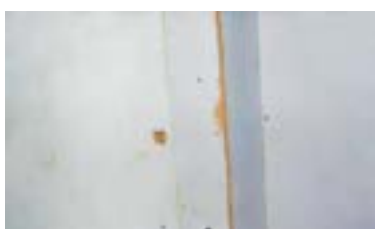
Figure 24 Chrysotile paper on fibreboard boxing
