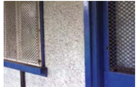
Figure 33 Chrysotile pebble-dash exterior wall coating
