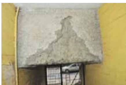
Figure 8 Sprayed coating on building passageway
