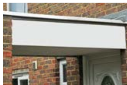
Figure 15 AIB panel in porch
