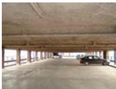
Figure 7 Sprayed limpet on car park roof
