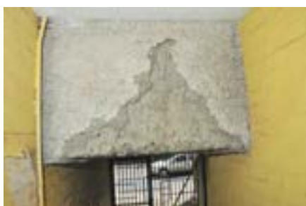
Figure 8 Sprayed coating on building passageway
