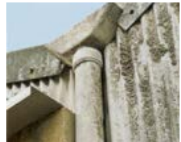
Figure 35 Asbestos cement downpipe
