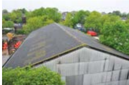
Figure 32 Asbestos cement roof and cladding
