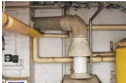
Figure 34 Asbestos cement boiler flue
