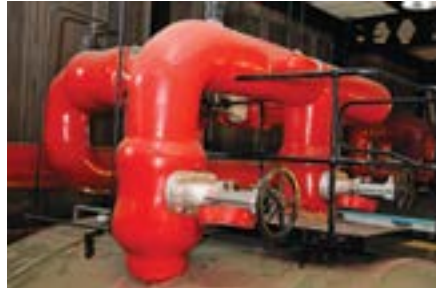
Figure 48 Asbestos-insulated supply pipes
