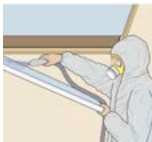
Figure 7.13 Spraying AIB
