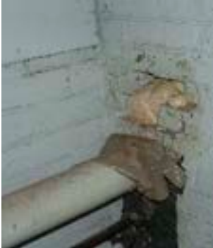
Figure 6.4 An enclosure sealed with expanding foam
