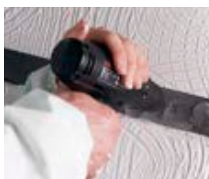
Figure 7.7 Textured coating being drilled through paste
