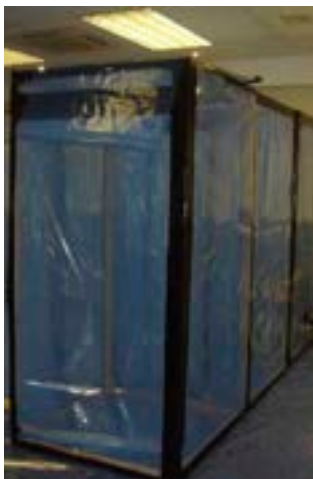
Figure 6.12 Flap arrangements for airlocks
