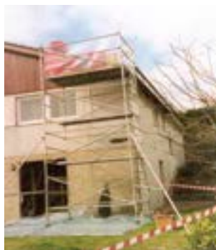
Figure 6.2 Work without an enclosure
