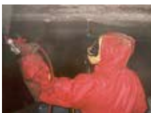
Figure 1.6 Controlled removal of asbestos
