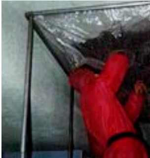
Figure 7.17 A sprayed asbestos coating being removed using a specialised glovebag within a traditional enclosure (the dark area is where the asbestos has been removed)
