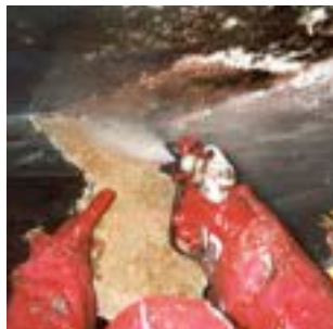
Figure 7.15 Spraying thin coating
