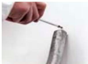
Figure 7.5 Shadow vacuuming during unscrewing of board
