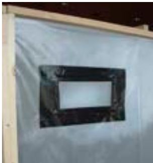
Figure 6.17 An enclosure being smoke tested
