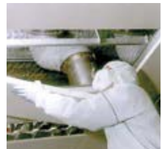
Figure 10 Removing panels to gain complete access for a Type 3 survey
