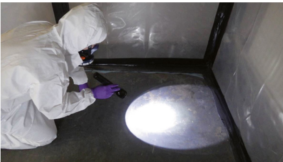
Figure 6.4 Analyst carrying out the thorough visual inspection
