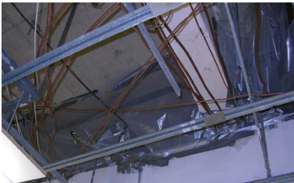
Figure A5.4 Void photo showing locations and extent of surfaces, cables and other items that need to be visually inspected for dust and debris
