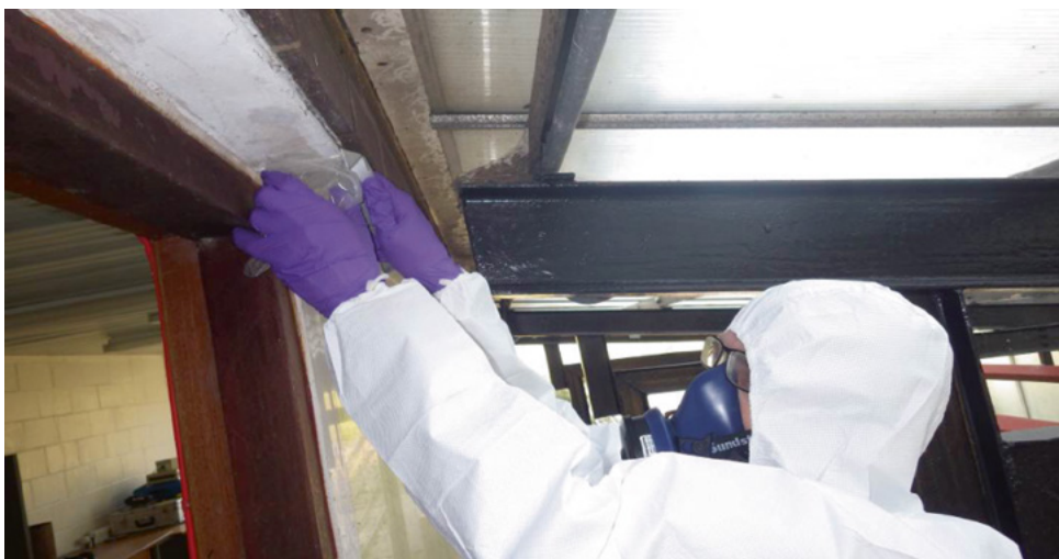
Figure 4.3 Sampling of AIB panels
