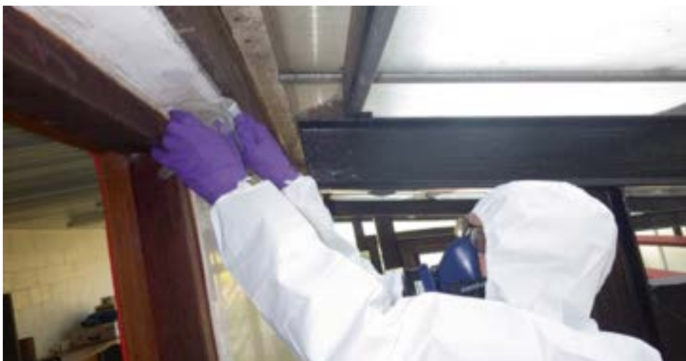
Figure 4.3 Sampling of AIB panels
