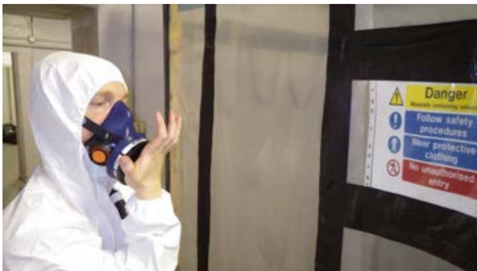
Figure 8.2 Pre-use wearer seal check (fit check) of half-face mask
