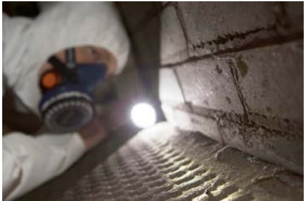
Figure 6.2 Analyst carrying out a detailed visual inspection
